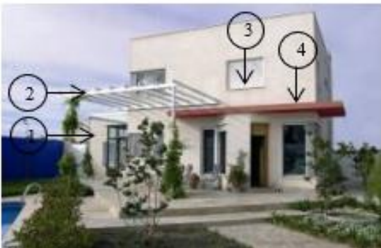
Photo 8: South and east prospect
