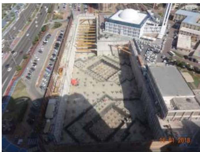
Figure 13 Final View of shoring system in place
