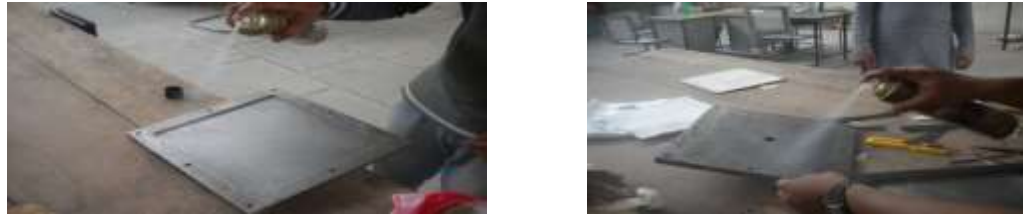
Fig. 4.3 Applying Silicon Spray
